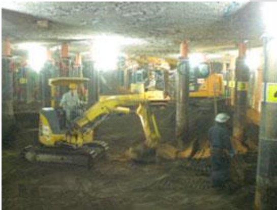
Below-floor excavation work
