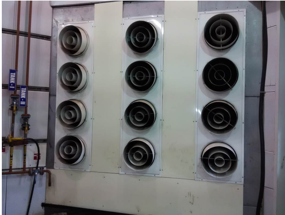
Fig 3.4 Inlet blower System
