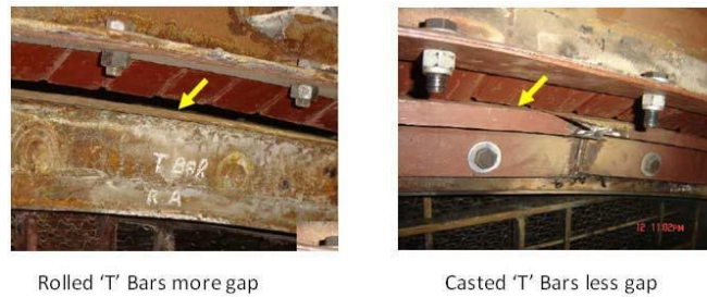
Figure 7: Reducing gaps by casted T-Bars
