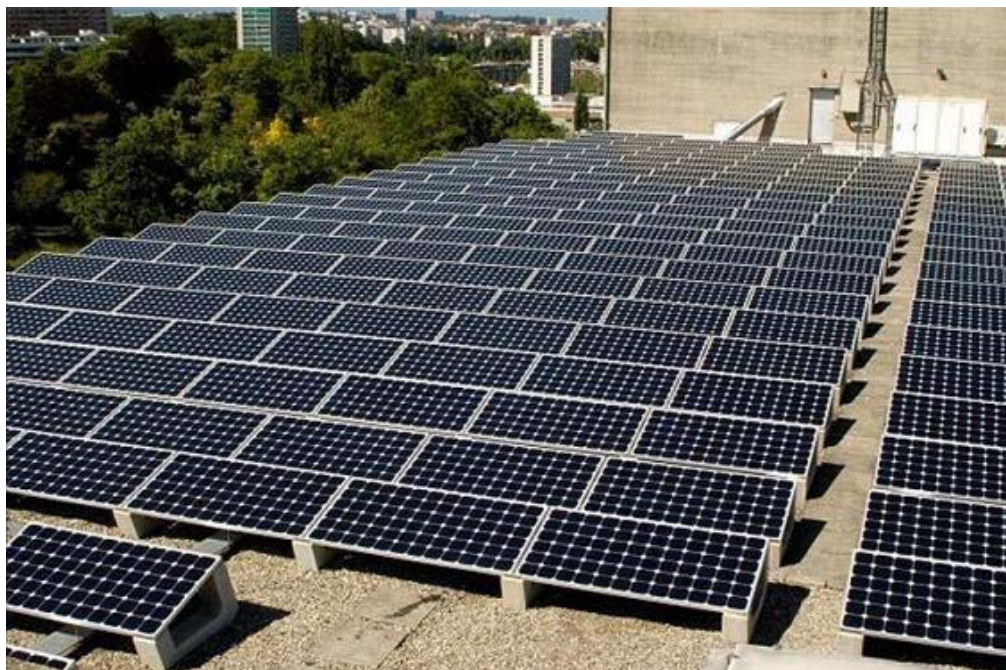
Figure 4: The rack design accepted for energy optimization
