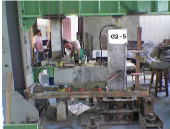
Fig.(10): Crack pattern and mode of failure for Specimen (5)
