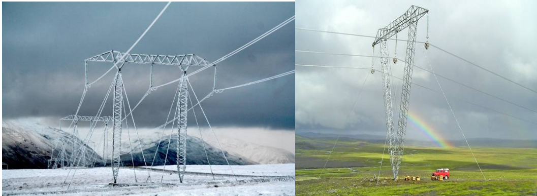
Fig 5.1 Guy wire attachment in a guy tower
