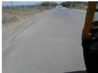
Fig.3 Urban road condition
