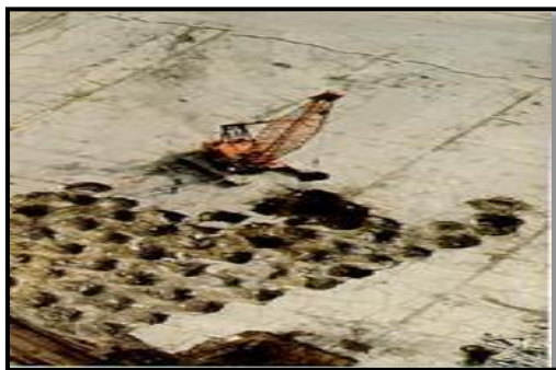
Fig-3 Deep dynamic compaction
