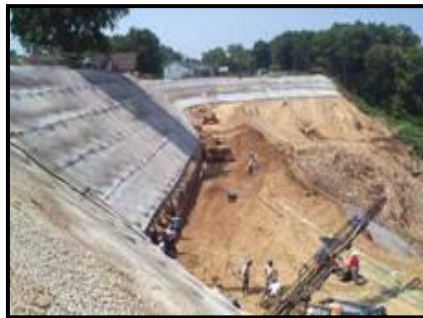
Fig-14 Soil Nailing
