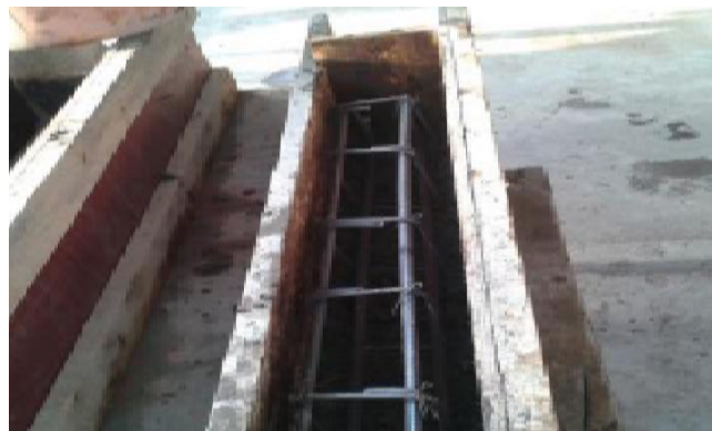
Fig 2 Casting of RC Beam.
