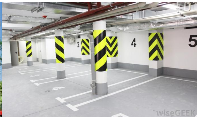
Figure 2: showing use of Soft storey in buildings
