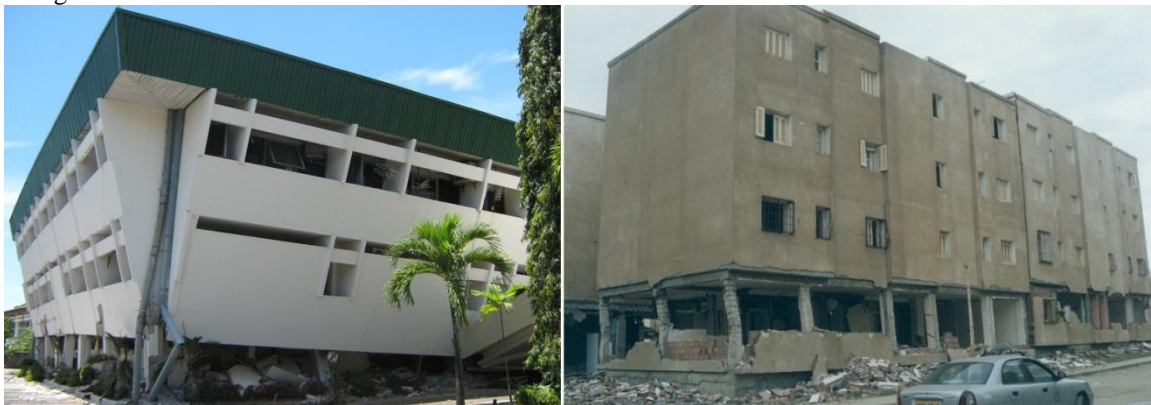
Figure 5. Failure due to large lateral displacement in soft storey
