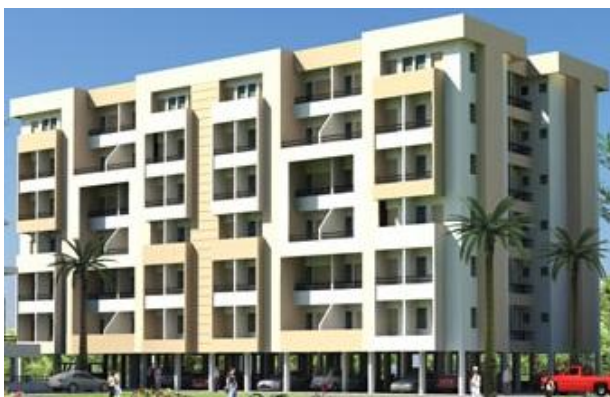
Figure 1: Soft storey buildings
