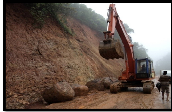
Fig. 6. Core stones in granite saprolite
