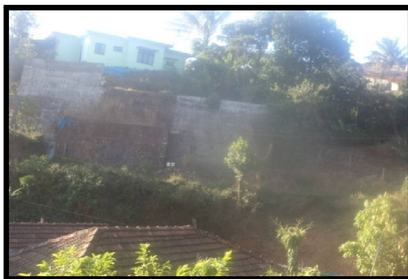
Fig. 8. Retaining wall – earth retention system in Mercara town
