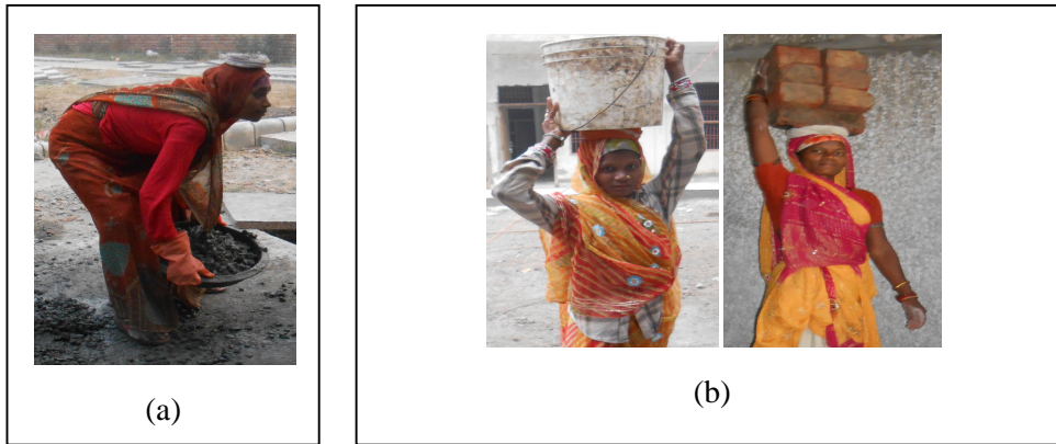
(a) Posture adopted during lifting headload (b) Posture adopted during carrying headload
