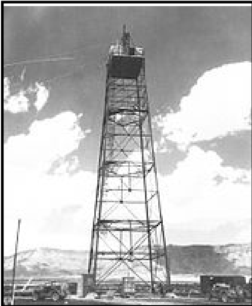
Fig.30 The 100-foot Tower on top of which the Gadget will be exploded
