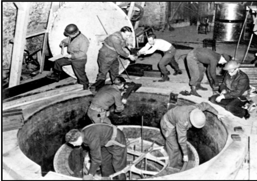
Fig.18. The last German experimental Reactor which failed
