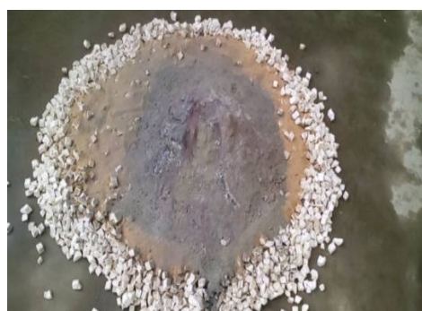
Thermocol concrete mixing
