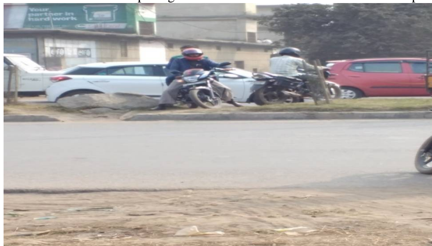
Fig. 5 (a) Unauthorised Openings (Source: Site visit photography)
