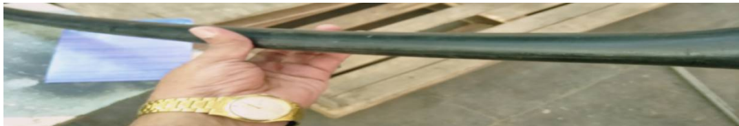
Fig. 5 Deformed Composite Pipe I
