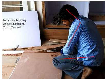
Figure 4: Worker applying veneer in awkward body posture.
