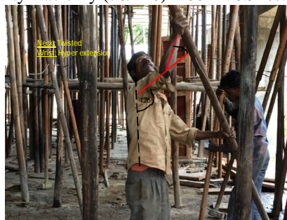
Figure 2: Worker removing Centering plates in awkward body posture.
