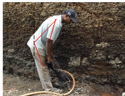
Figure 1: Worker doing excavation in awkward body posture.
