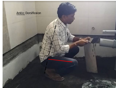
Figure 3: Worker doing tiling work in awkward body posture.
