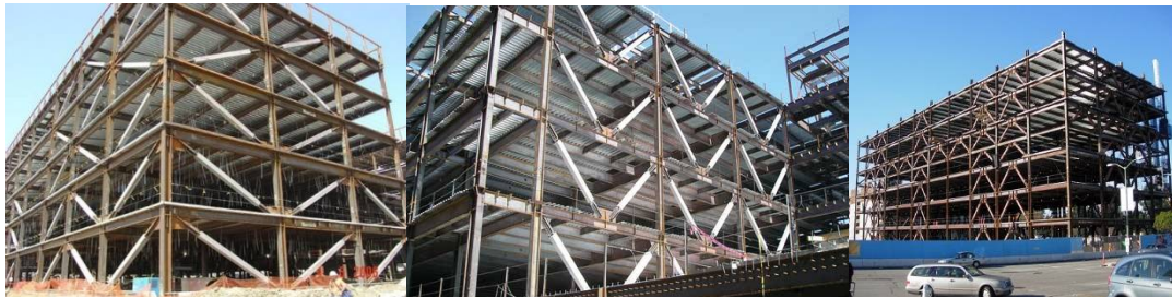
Fig 1: Braced Frame Structures
