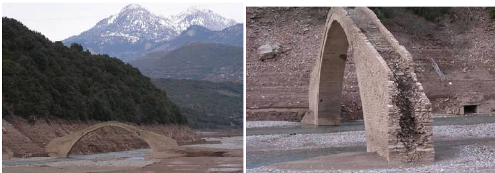
Fig. 21,22. The Manolis bridge after a protracted drought 03/01/2007
