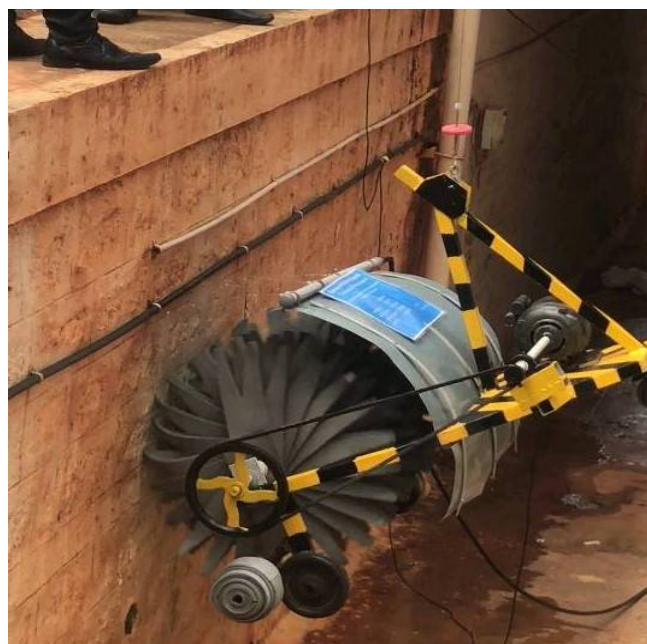
Figure 6 Façade cleaning in progress
