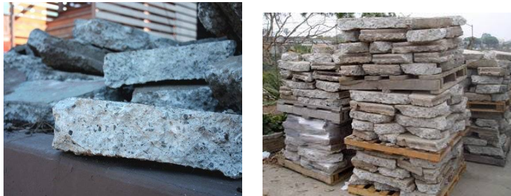
Figure 10: Material storage for reclaimed granite, concrete and yellow stock bricks on the Olympic Park
