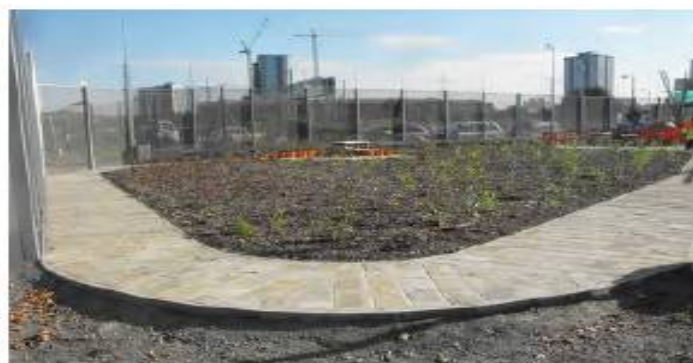
Figure 12: Repurposed concrete for walkway pavement
