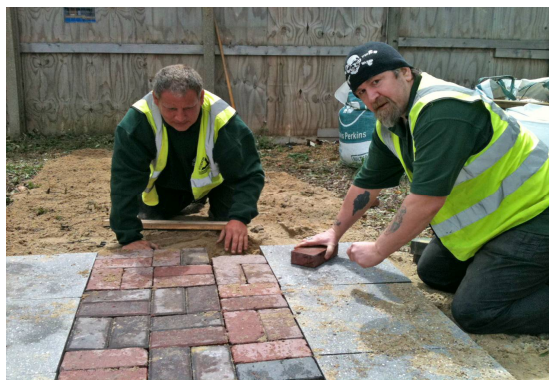
Figure 11: Repurposed concrete for floor paving at Construction Zone A
