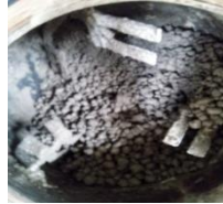
Fig 9 :Mixing in drum mixer
