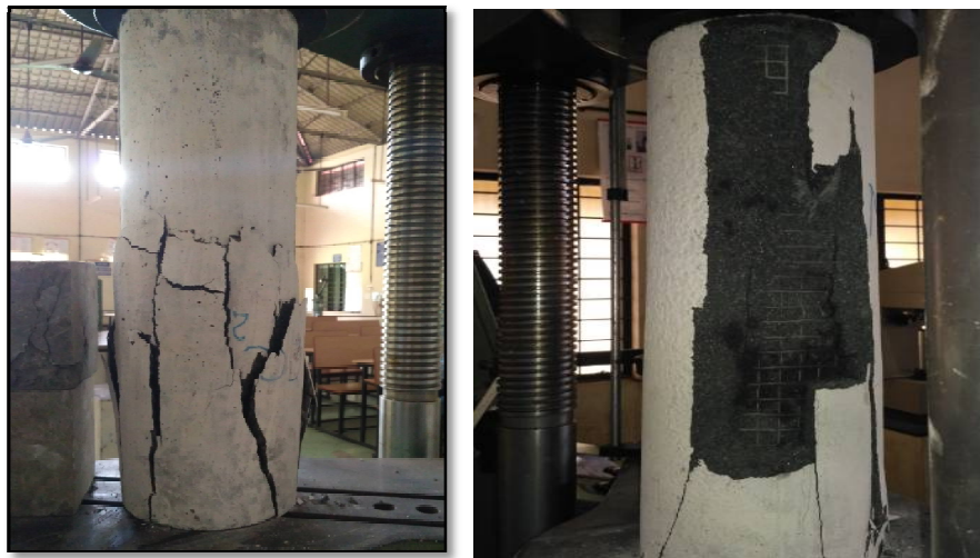
Fig.10. Crack pattern of Jacketed Columns (a) Concrete Jacketed column (b) Micro concrete jacketed column
