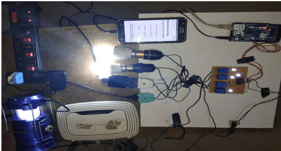
Figure 6 Home automation System
