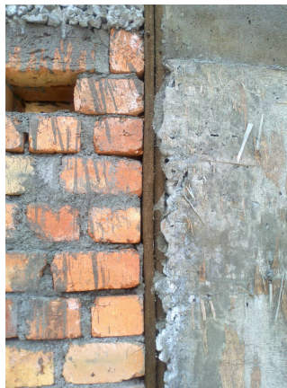
FIG.12.EXPANSION JOINTS USING BITUMEN PADS.
