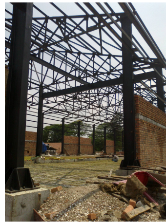
FIG.11.SUPPORTING PILLARS OF GODOWN
