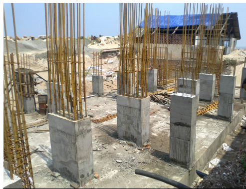
FIG.1 THE ON GOING CONSTRUCTION OF WET TABLE FOUNDATION AT MS PLANT
