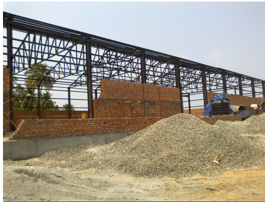
FIG.5.CONSTRUCTION OF STORAGE GODOWN
