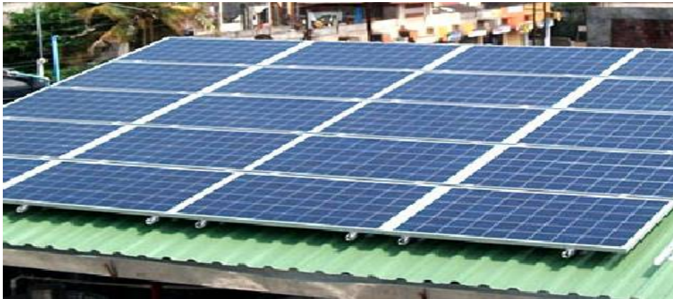
Fig-2: Solar PV plant installation on domestic sheeted roof top.
