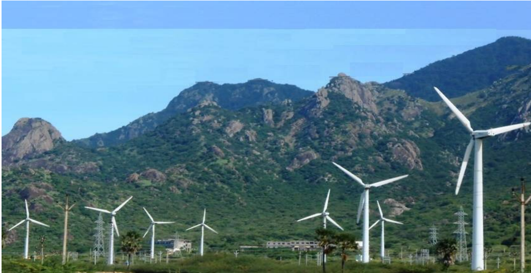
Photograph (1): Wind fan installed on Sea level.
