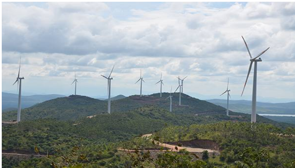
Photograph (2): Wind fan installed on above Sea level.
