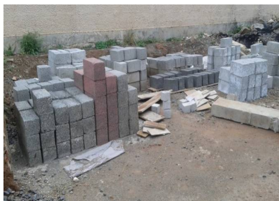
Fig.19:Curing of Cinchona Ash concrete Blocks
