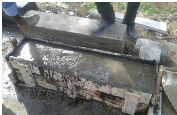
Fig 4 Applying on the concrete and vibrating the mould
