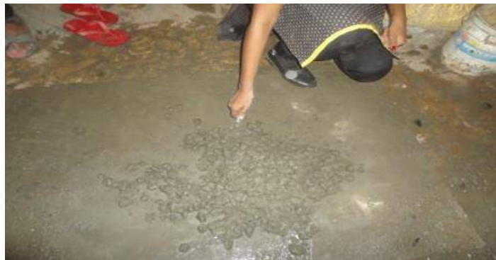
Fig4.Hand mixing
