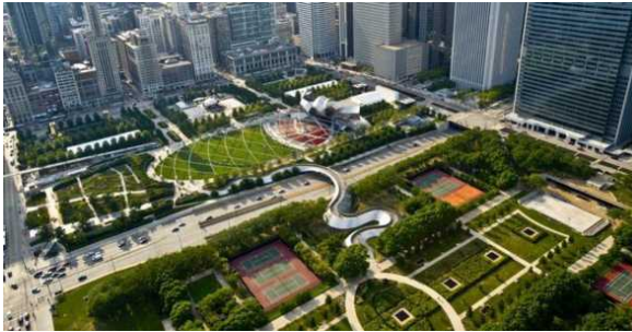
Figure 2 Showing Hamilton Green Roof
