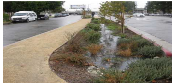
Figure 5 Showing the installation of vegetated Swales
