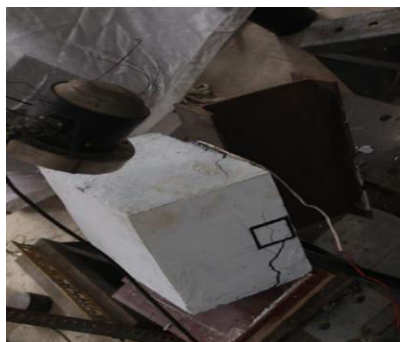
Fig 12. Failure of square connector specimen
