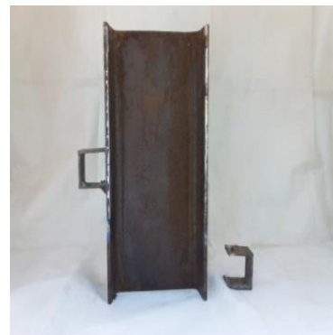
Fig 13. Part of fractured square connector attached to the steel beam
