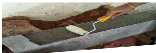
Fig: 5. Application of Epoxy Resin on the Surface of the Beam
