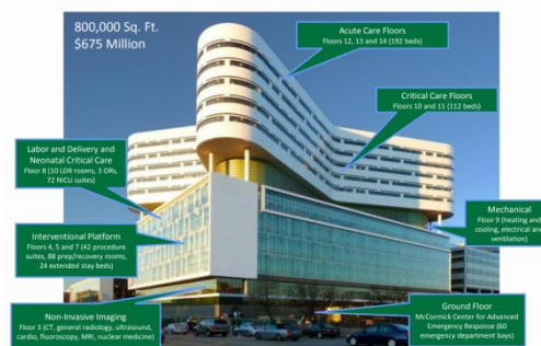
Figure (8): Departments of the Tower in Rush Hospital
