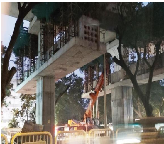
Figure 3.5: Construction activity near road.
