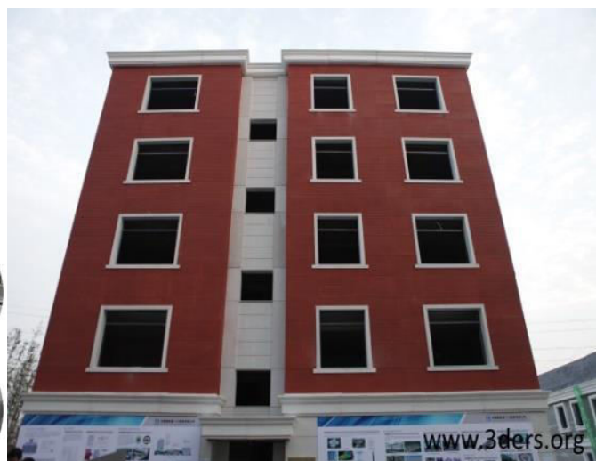
Fig 2.2 WinSun China build world's first tallest 3D printed apartment building
