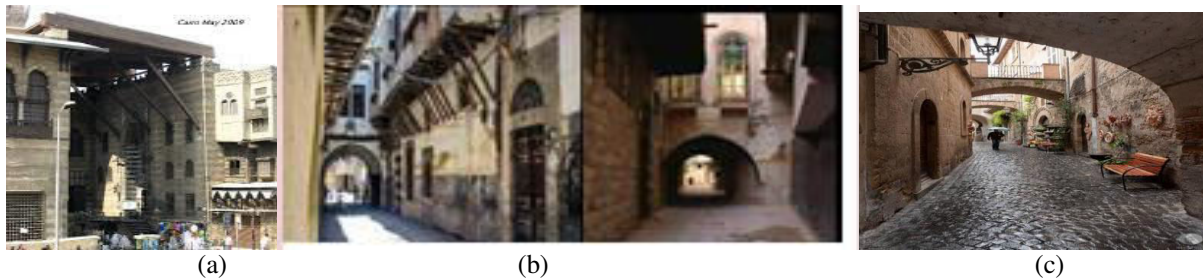
Fig.7: Coverage in cities of an Islamic character: (a). Flat against the roofs in Andalusia (b), where brick vaults and two thresholds of wood and grapes were used, while Aleppo used stone cellars (c) 7 .
