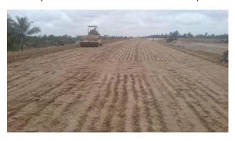
Figure 1 Showing cement stabilised subgrade at test site
