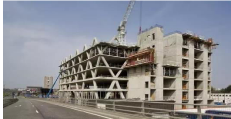
Fig 1.1: Bracings are placing in the building
