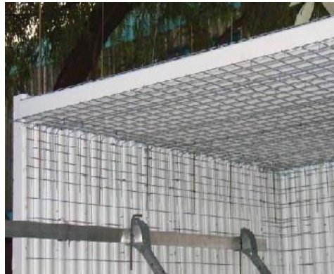
Fig 3.8 Wall panel hold vertical before plastering
