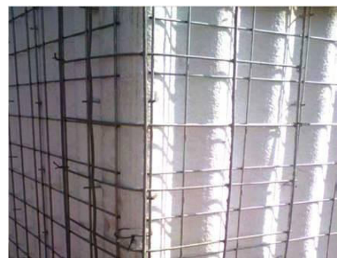
Fig 3.7 Exterior wall joints
