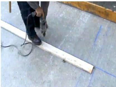
Fig 3.2 Position of panel mark
