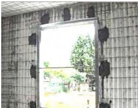
Fig 3.9 EPS Door/Window hold
