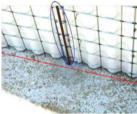
Fig.3.4 EPS Core panels between the starter bars
