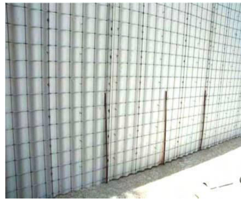
Fig 3.5 Overlapping mesh starting from a corner
