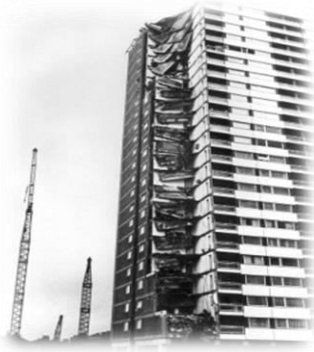
Figure 1(a)- Ronan point building after 16 May 1968.
