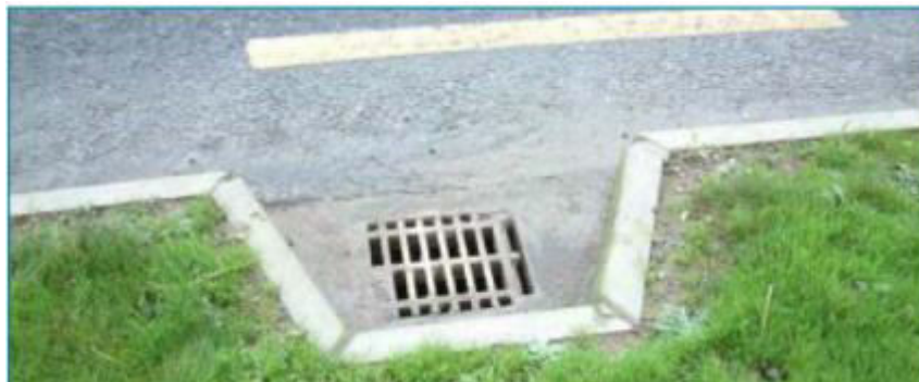
Fig 1: Kerbs & Gully (inset into verge)
