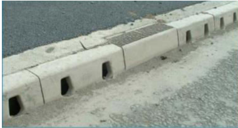
Fig 3: Combined Kerb and Drainage Block
