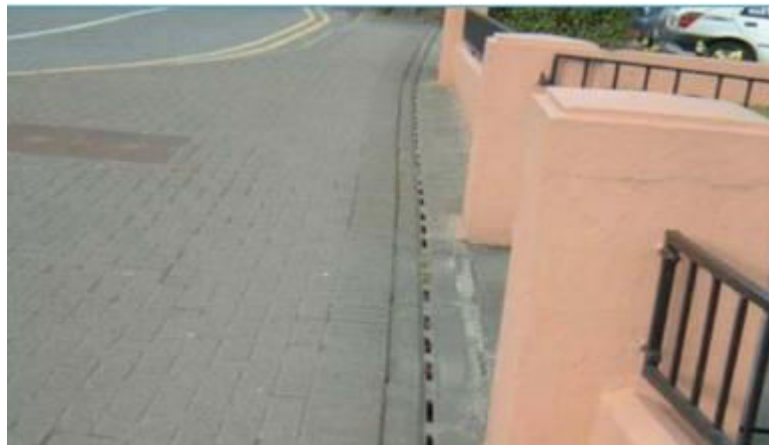
Fig 4: Linear Drainage Channel
