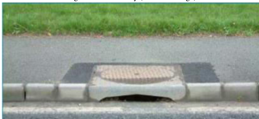
Fig 2: Side Entry Gully
