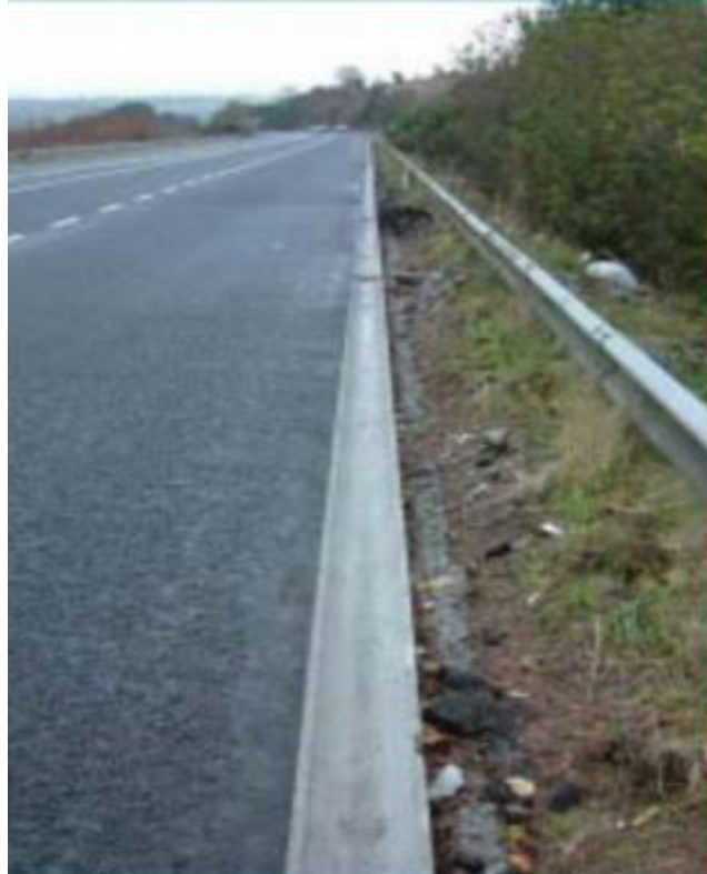
Fig 5: Surface Water Channel
