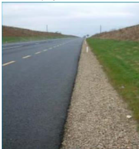
Fig 6: French Drain
