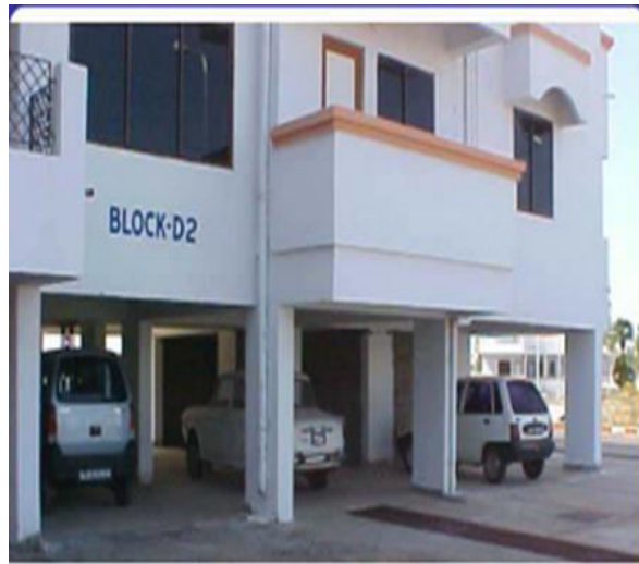
Figure 1.1 Vertically irregular buildings. (a) OGS Building (b) Stepped type building
