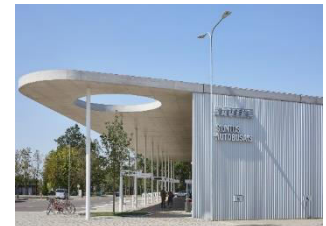
Figure 12. Corrugated aluminium wall and steel columns Source: Author
