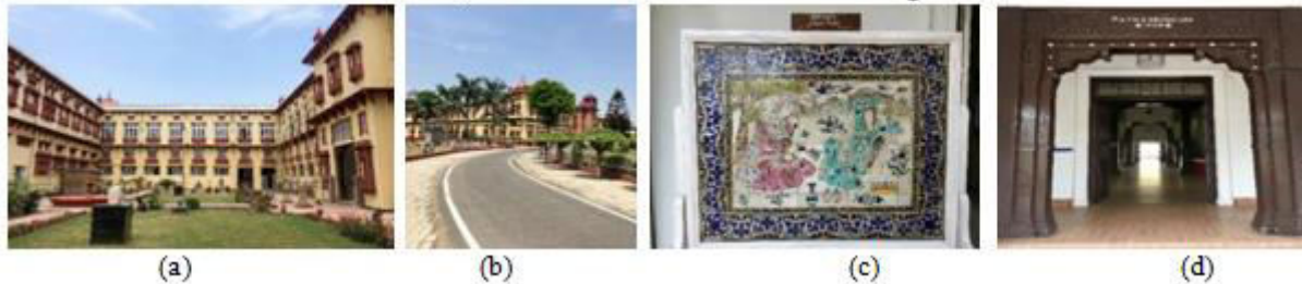
Figure 3 (a), (b), (c), (d) Images showing Patna Museum and the inside of Patna Museum.
