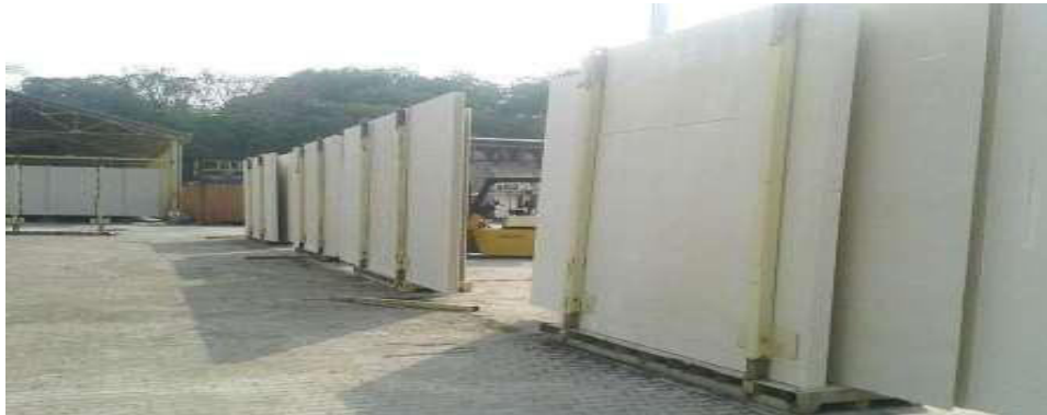
Fig.1.1 Panels in stillages
