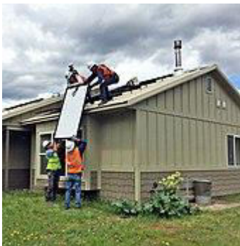
Workers install residential rooftop solar panels
