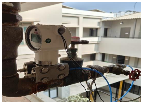
Fig. 4. Pressure transmitter in the tank outlet.
