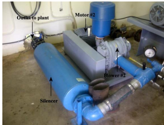
Fig. 2. Inside of the blower house, showing blower #2 and the air outlet pipe leading to the treatment plant
