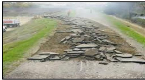
Fig:1 Demolished Asphalt Pavement
